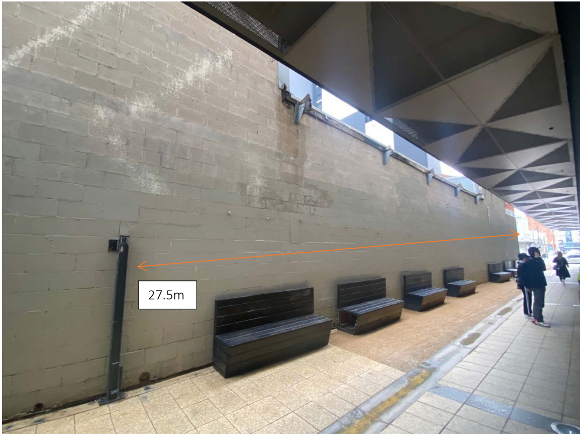
fig. 2 The wall in its current condition
