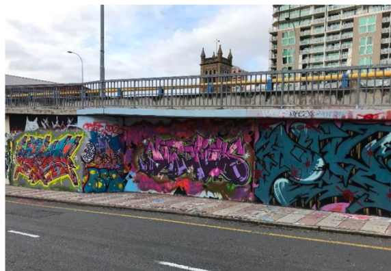
Morphett Street bridge opposite FIP
